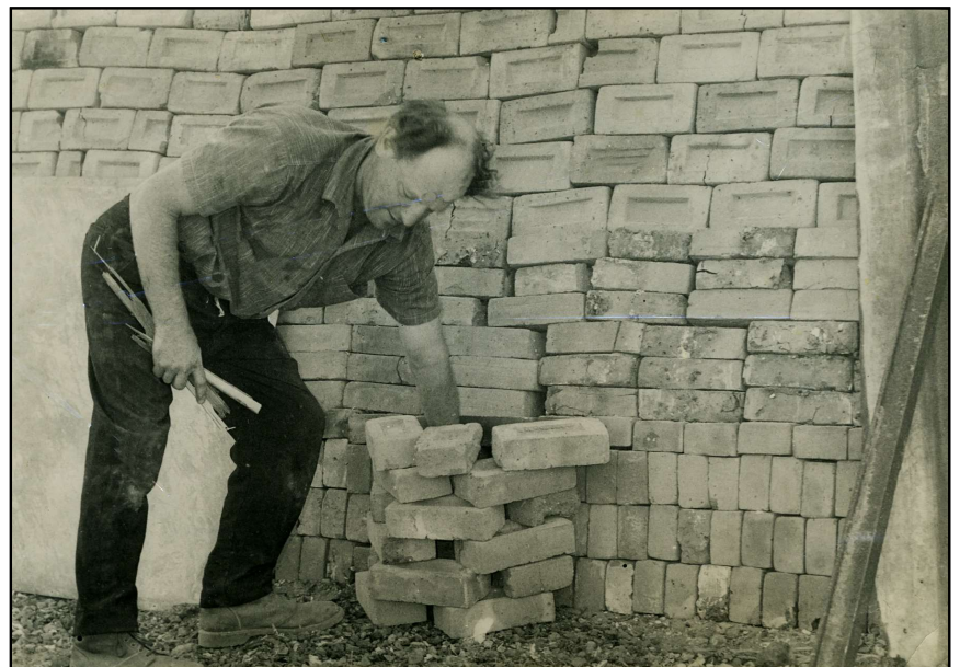
4.7 Noel Pycroft lights the clamp – photograph taken in 1950.
