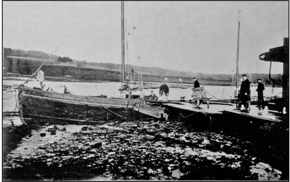
Loading bricks onto the barge "Langstone" for delivery along the coast.
